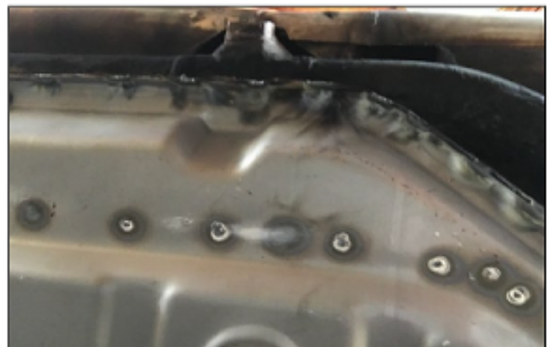
Underside shot of floor pan replacement piece.
