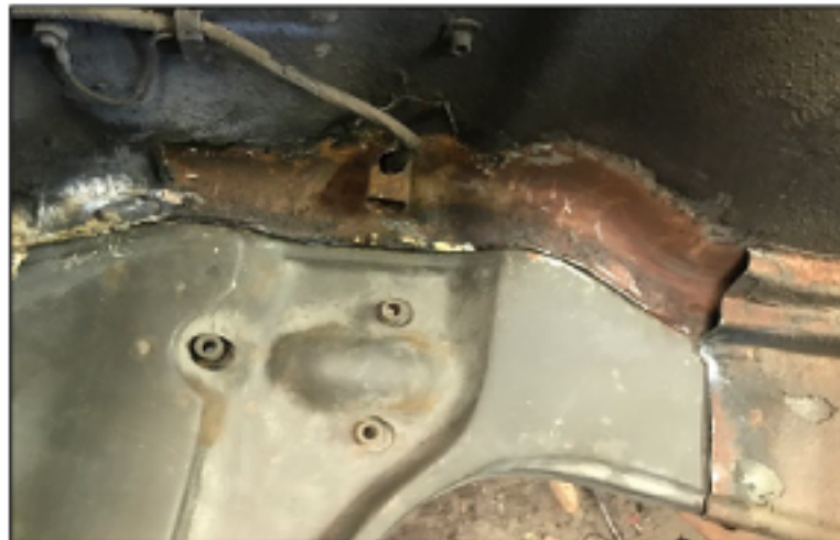
Opposite side from the battery where the area is not as rusted compared to the battery side so it didn't need to be replaced.
