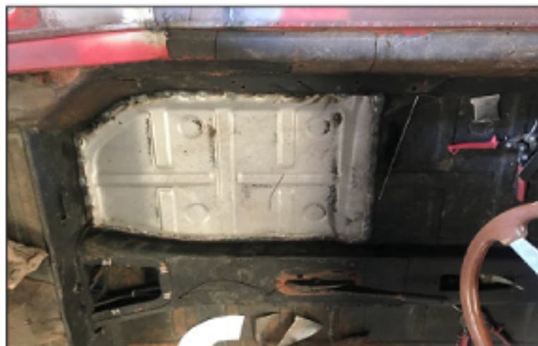
Looking down through the open top to the driver's side floor pan that had a rectangular piece cut out of it
